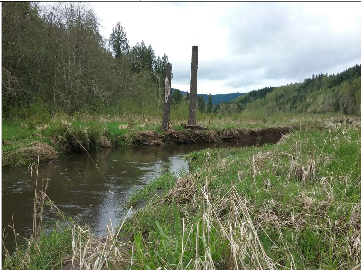
April 2019 – Post-Construction and Planting
