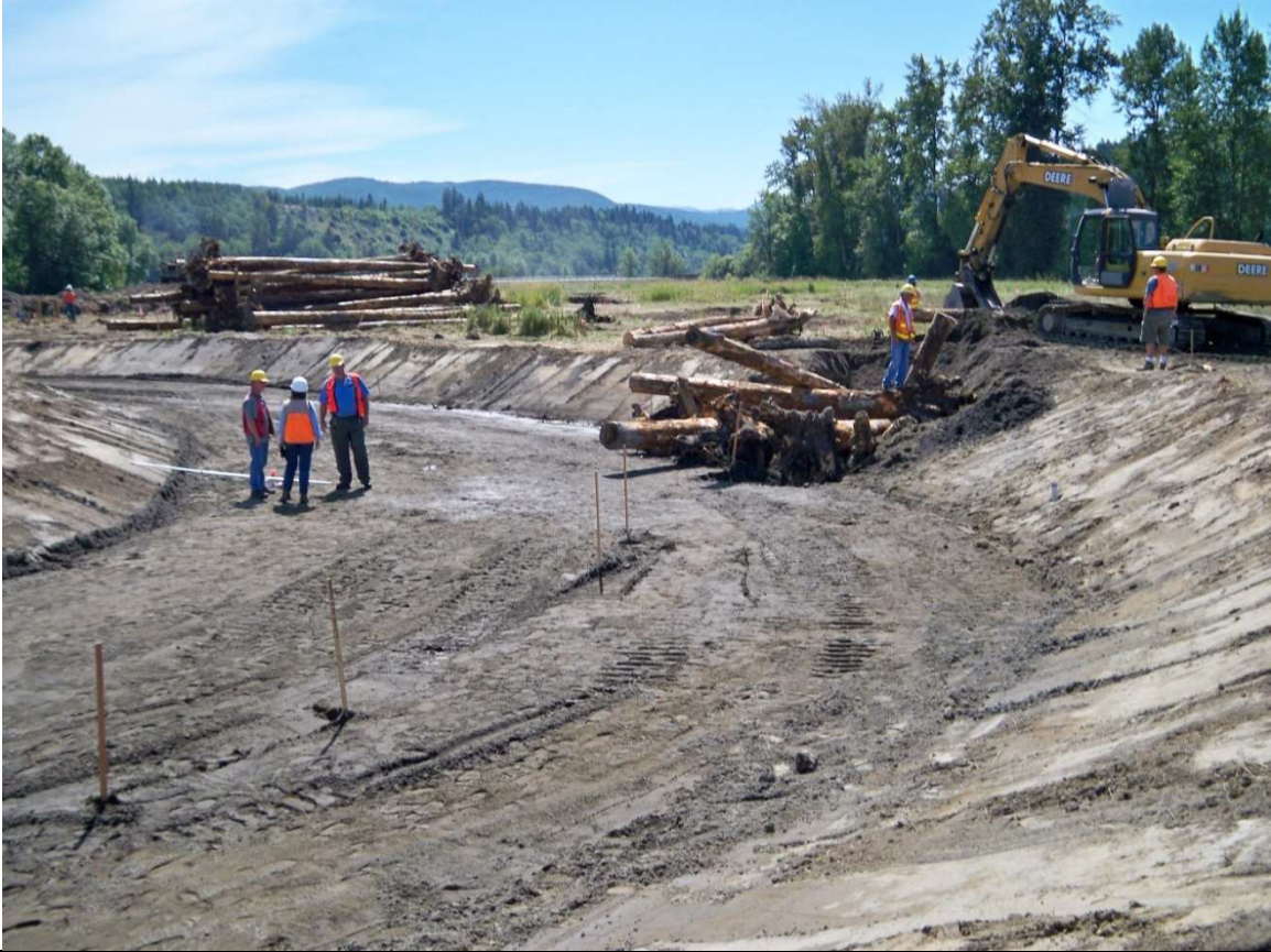
July 2009 – During Construction
