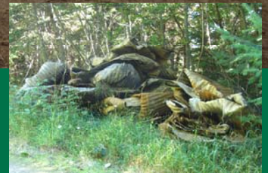
The Land Trust has begun road decommission on former industrial timberland acquired in 2009, located near the Mount Rainier National Park. Culverts (right) were removed and the road bed was roughened to speed revegetation.
