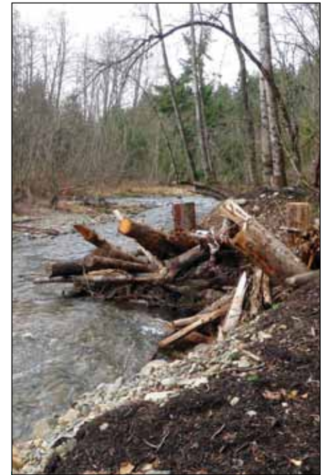
Over 40 salmon-friendly engineered logjams, like this one have been installed on Land Trust and Eatonville properties along the Mashel River by the Nisqually Tribe and the South Puget Sound Salmon Enhancement Group.
