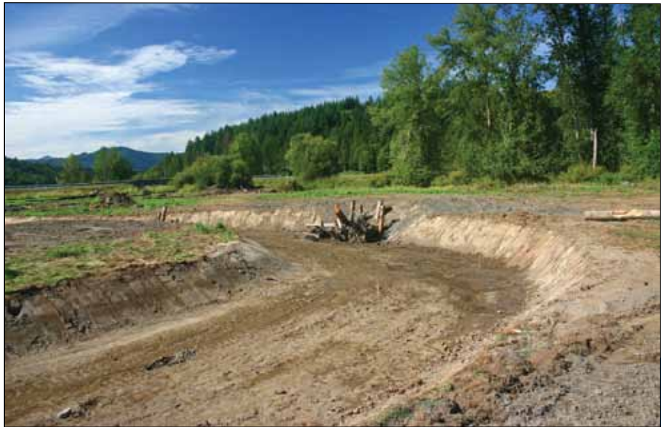
This newly dug channel will restore meanders to Ohop Creek. Forty-two engineered logjams like the one above will provide salmon-friendly pools.
