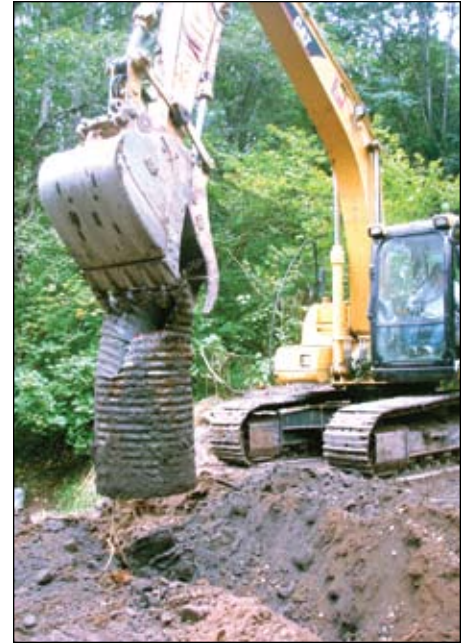
Three rusted metal culverts blocked salmon passage into the largest off-channel wetland complex on the Nisqually River
